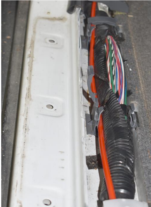
Wiring loom faults in vehicles can be very difficult to locate
